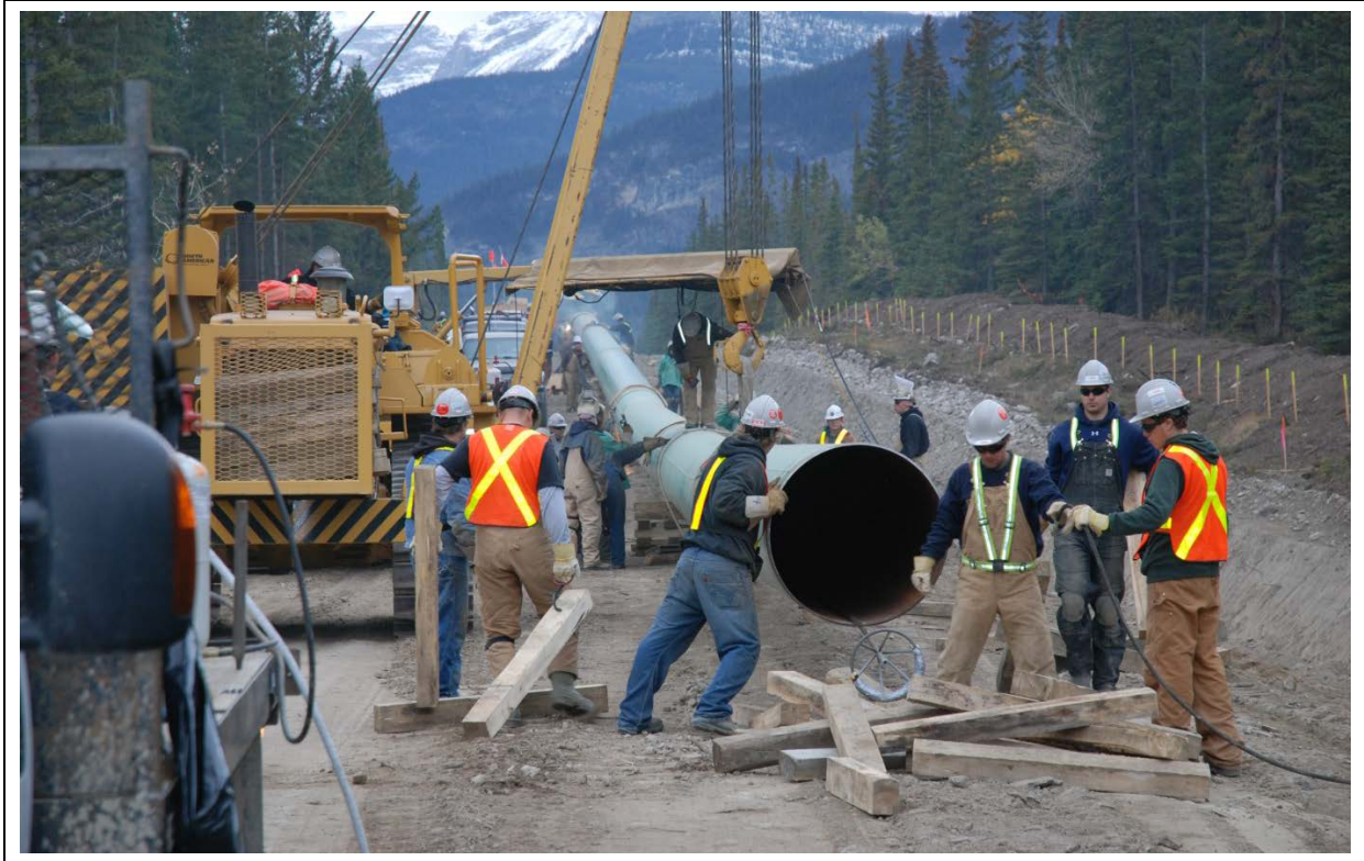
Plate 2.1.1 Typical Pipeline Construction
