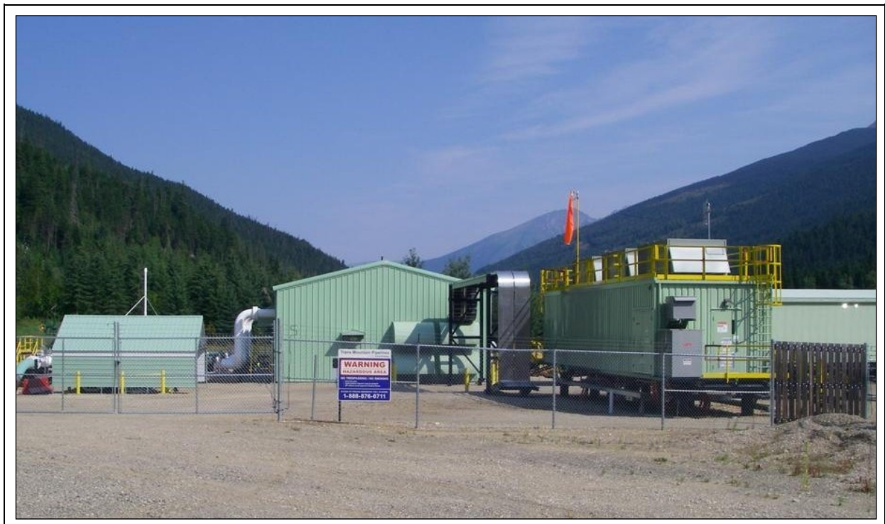
Plate 2.2.1 Typical Pump Station (Chappel)
