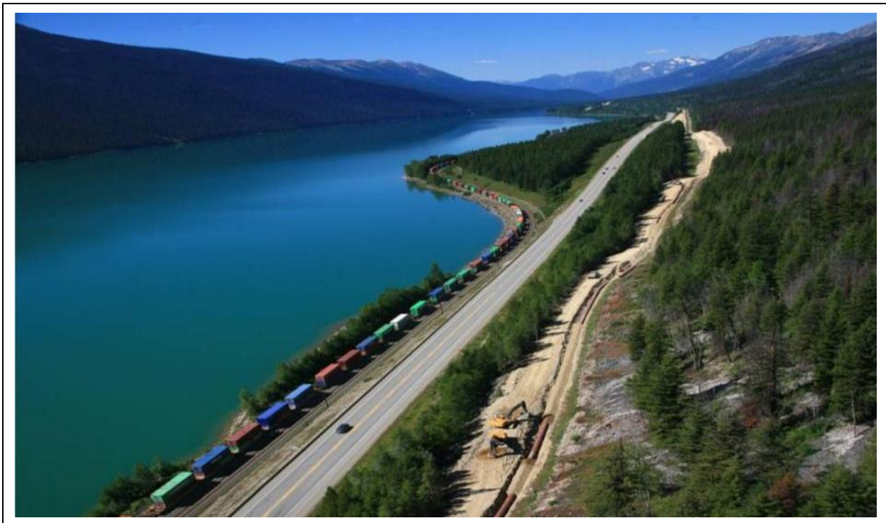
Plate 2.4 Construction of Trans Mountain Expansion Anchor Loop in Mount Robson Provincial Park
