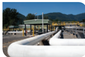
Sumas Pump Station and Terminal
