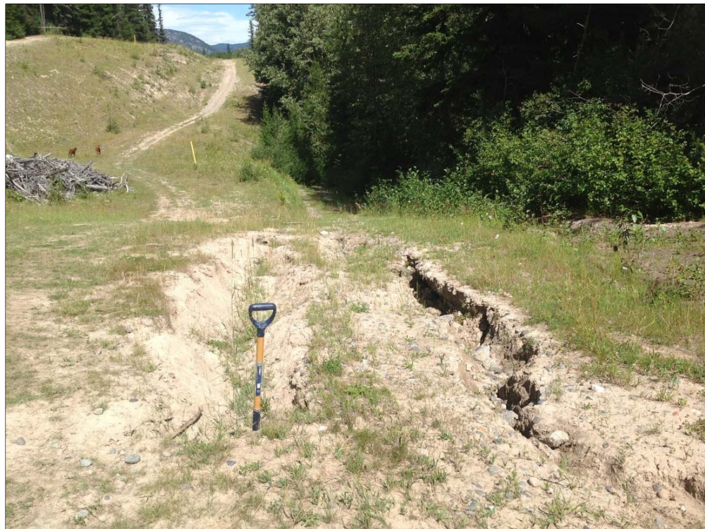
Photograph 5-4. Surface erosion in fine textured glaciolacustrine sediments along the ROW at RK 982.7
