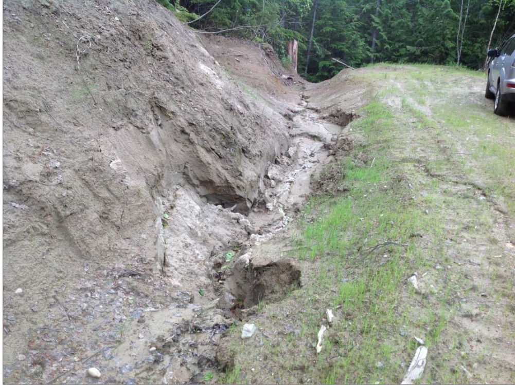
Photograph 5-1. Ditch erosion in fine sands near RK 571
