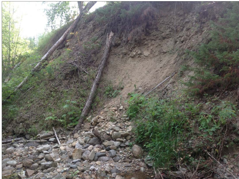
Photograph 5-3. Shallow debris slide on gully sidewall near RK 686.4
