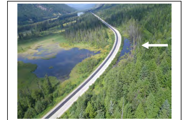
Plate 2 Overview showing riparian shallow open water (open water pond) (August 12, 2012).
