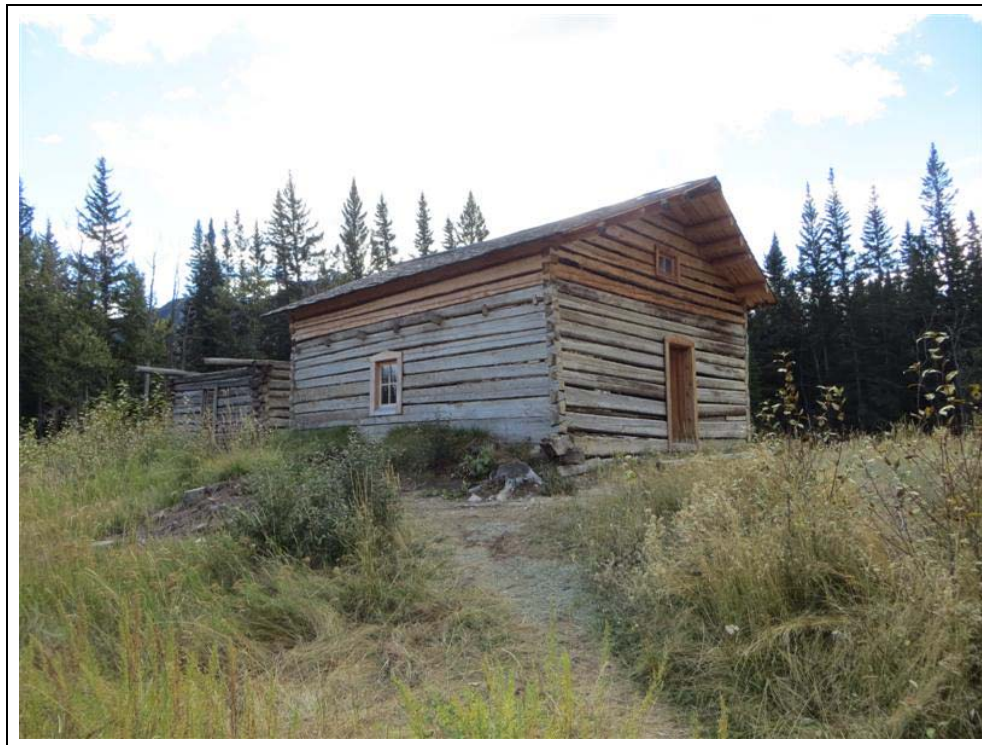
Plate 5.1.13-1 The Ewan and Madeline Moberly homestead built in 1908 (September 2013).
