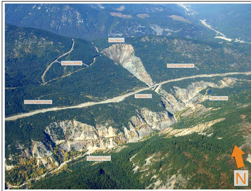
Plate 4 Existing TMPL right-of-way within Coquihalla Canyon in foreground and proposed corridor beside Coquihalla Highway and FOTS in mid-ground.
