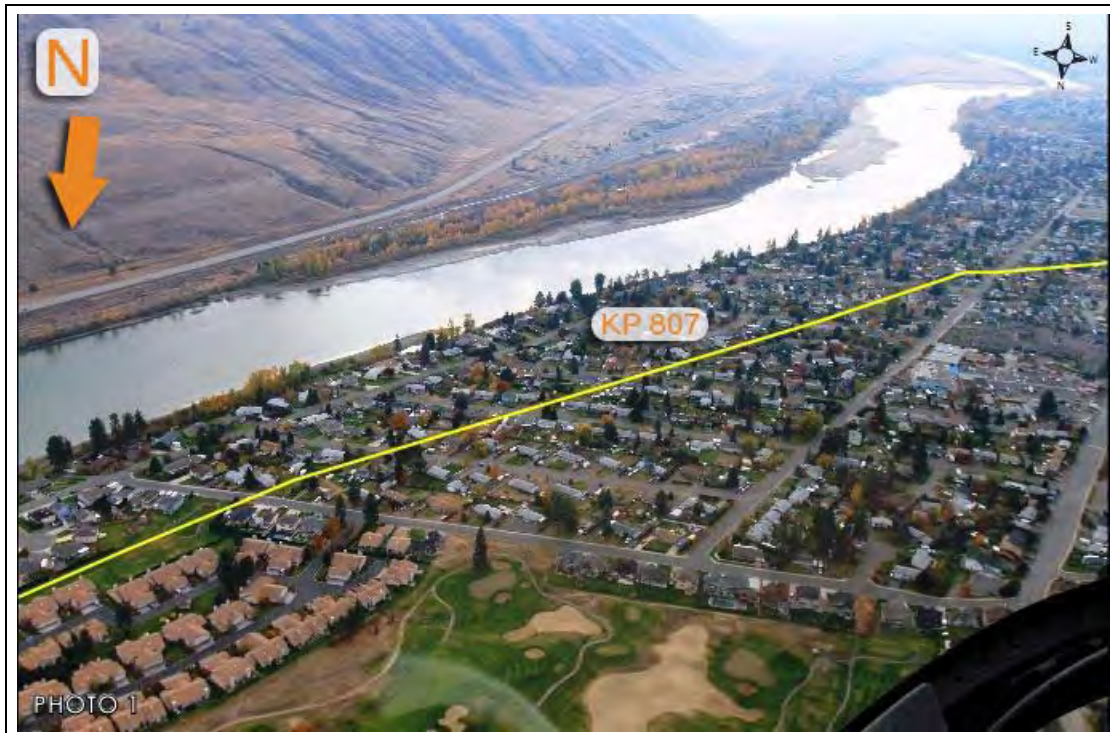
Plate 2 Existing TMPL right-of-way (shown in yellow) encroached by urban development through the community of Westsyde.
