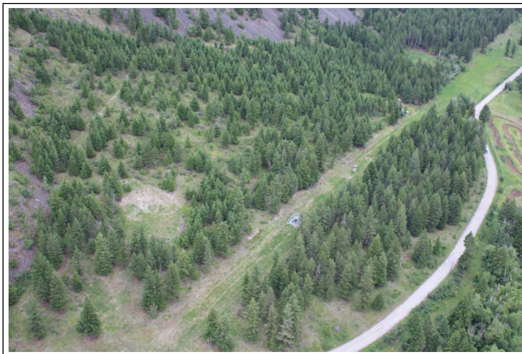
Plate 7 Aerial view of the proposed Black Pines Pump Station Site (May 27, 2013).
