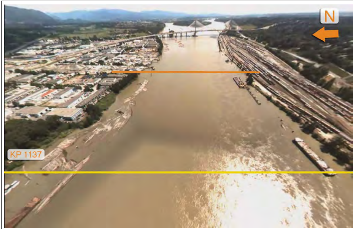
Plate 5 Overlooking the existing crossing of the Fraser River looking east with existing TMPL right-of-way (shown in yellow) in foreground, proposed pipeline corridor (shown in orange) in mid-ground and Port Mann Bridge in background.
