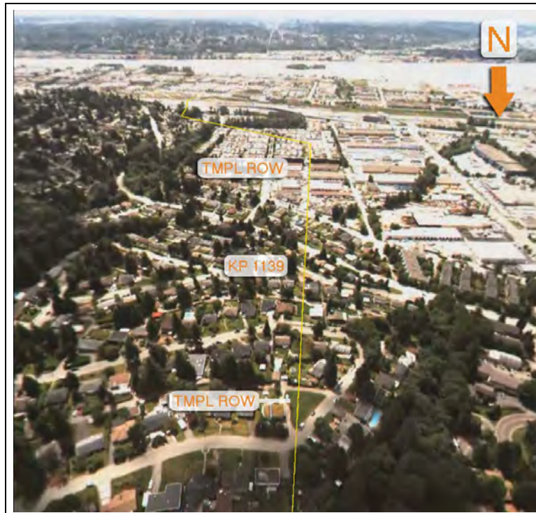
Plate 6 Looking south along the existing TMPL right-of-way (shown in yellow) encroached by urban development in the City of Coquitlam, BC.
