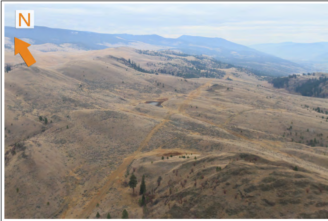
Plate 3 Existing FOTS right-of-way within Lac Du Bois Grasslands Protected Area.
