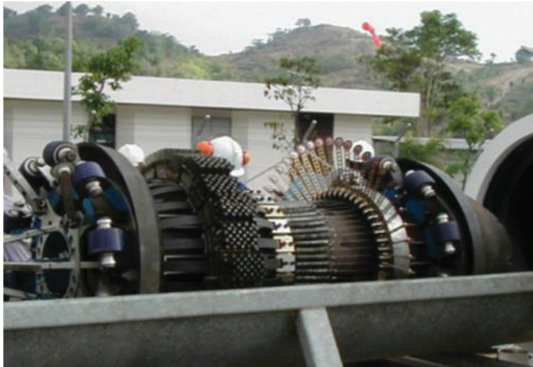
Figure 3: Image courtesy of BJ Pipeline Inspection
