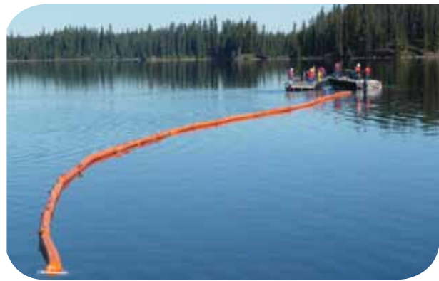
Exclusion boom is deployed across or around sensitive areas and anchored in place to deflect or contain approaching oil
