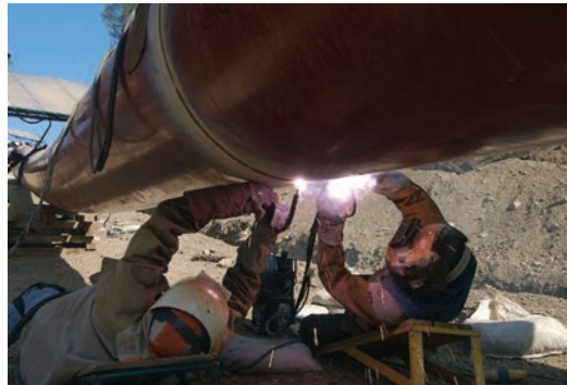
Figure 2: Image courtesy of TransCanada PipeLines Ltd.
