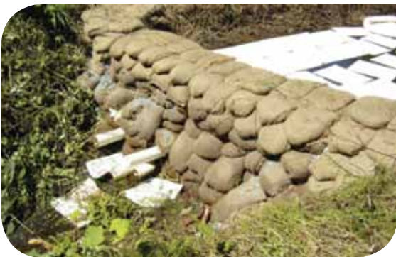
Inverted weir dam allows clean water to flow from the bottom so floating oil is blocked at the surface
