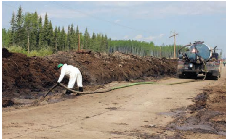
Figure 2: Workers use vacuums to clean up oil
