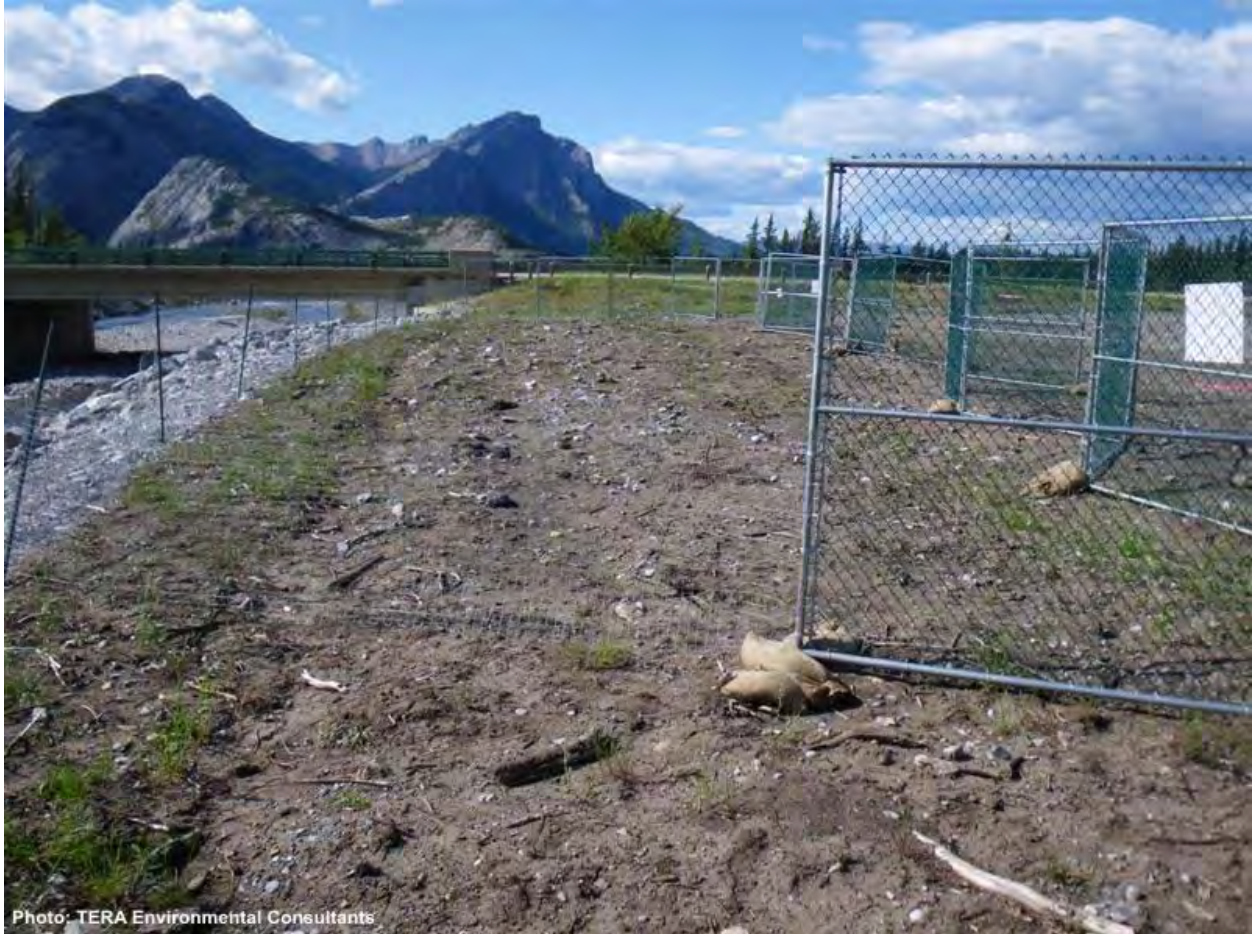
Figure 11. View of construction panel fencing being anchored with sand bags at a location know for high wind speeds. The majority of these fencing installations required no supplemental bracing or anchoring (June 2009).
