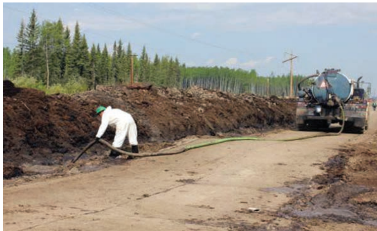
Figure 2: Workers use vacuums to clean up oil
