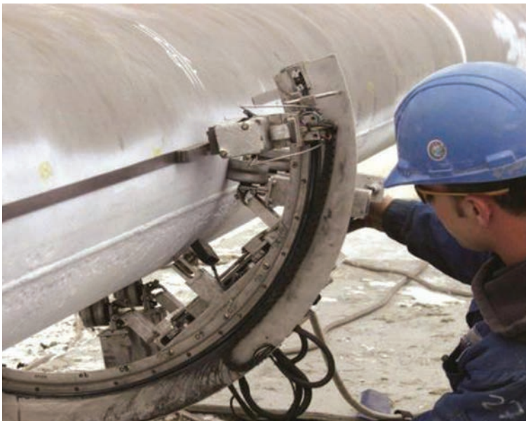
Figure 4: Image courtesy of BJ Pipeline Inspection
