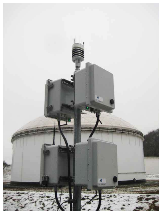
Ambient Air Monitoring Equipment at Sumas Terminal
