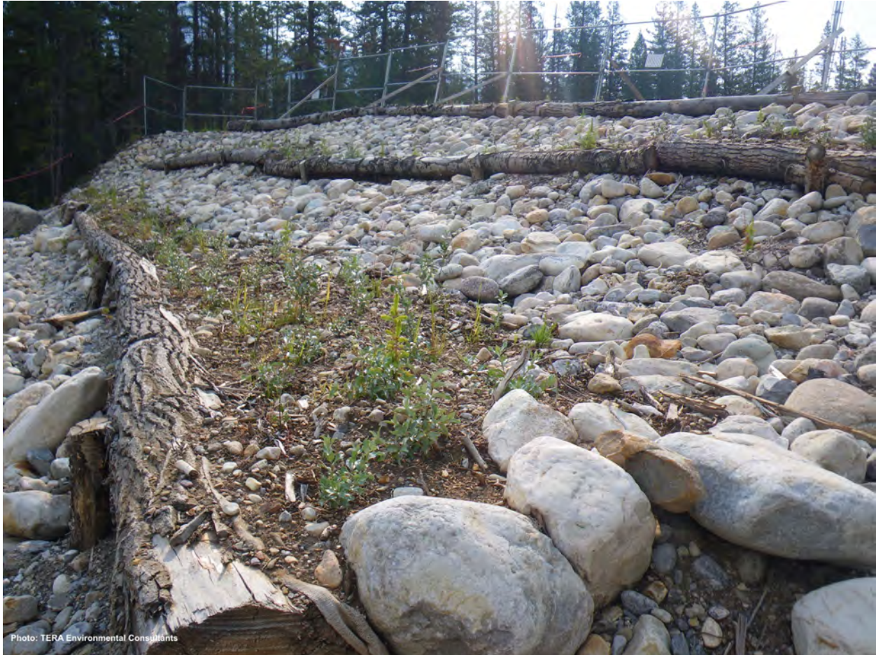
Figure 9. View of a riparian planting and woody plant material thriving behind a log retaining structure at Snaring River (August 2009).
