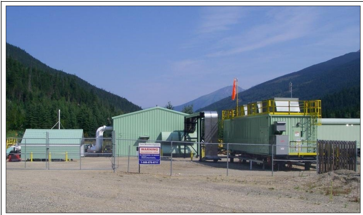
Plate 2.2.1 Typical Pump Station (Chappel)
