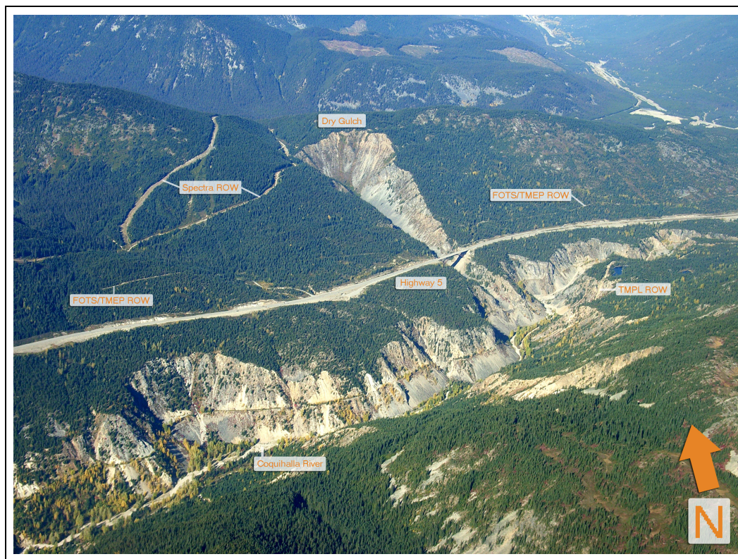
Plate 4.2.4 Existing TMPL easement within Coquihalla Canyon in foreground and proposed corridor beside Coquihalla Highway and FOTS in midground.
