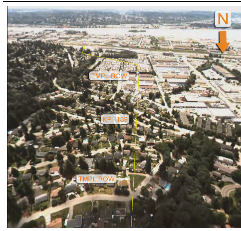
Plate 4.2.6 Looking south along the existing TMPL easement encroached by urban development in the City of Coquitlam.
