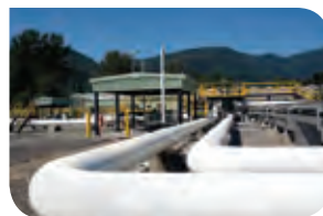
Sumas Pump Station and Terminal
